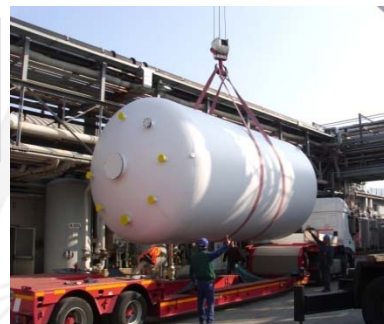
VERTICAL TANK Ø 3500 H. 7000 FOR SODIUM HYPOCHLORITE
